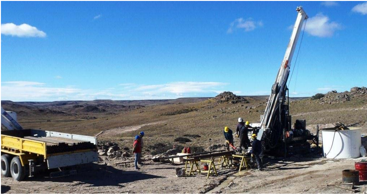
Photo 1: Current drilling at SM6
