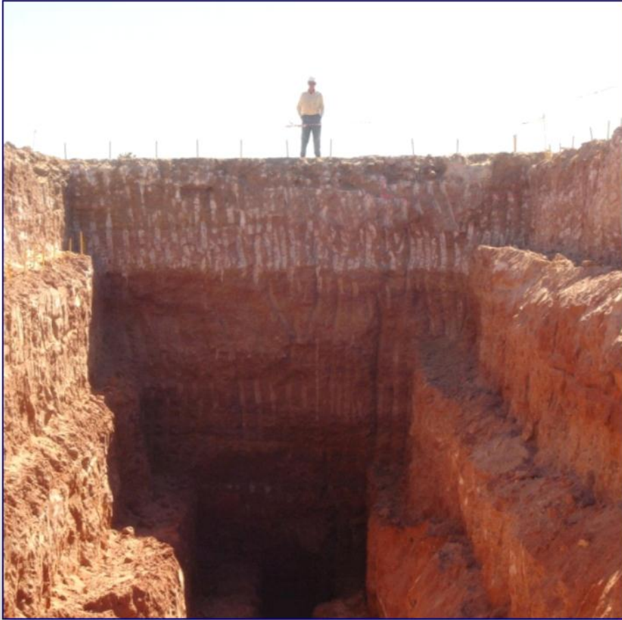
Trench for Bulk Sample
