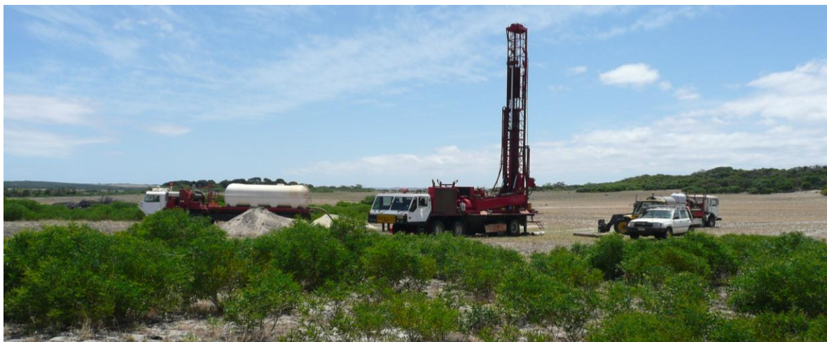
Photos of the baseline well being drilled on Eneabba's Sargon Tenement:-
