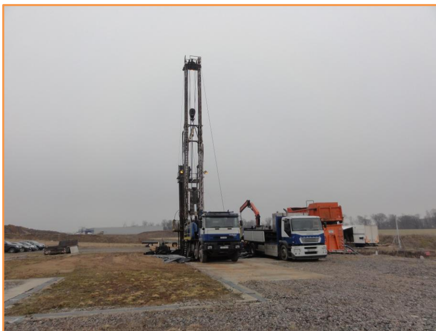
Figure 2 - Workover at Folschviller-2 well
