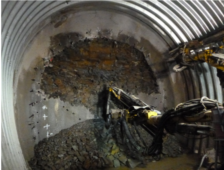
Commencement of construction of the underground exploration decline tunnel
