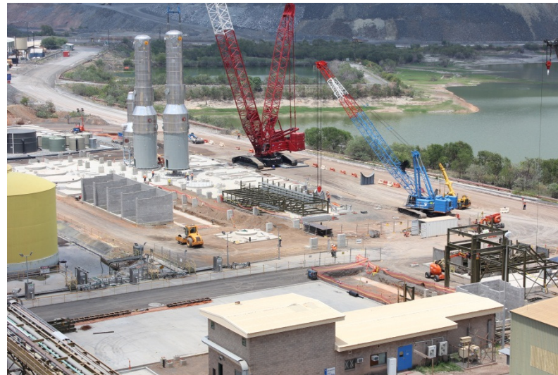
Construction site for Brine Concentrator
