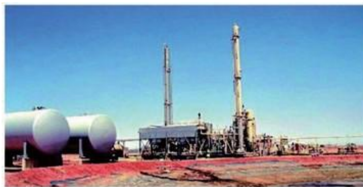
Eromanga Gas Plant, Australia
