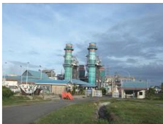
Sengkang Power Plant, South Sulawesi, Indonesia, initial CCGT 135 MW capacity (1997)
