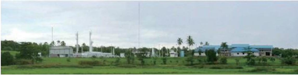
EEES Kampung Baru Sengkang, Indonesia Central Processing Plant (CPP)
