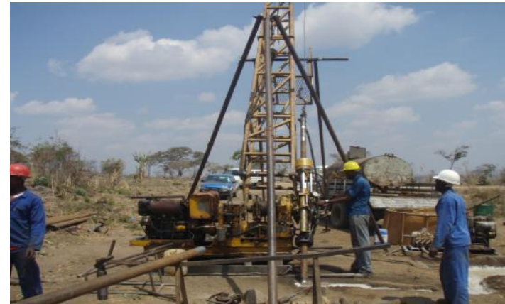
Drilling at Kanyika
