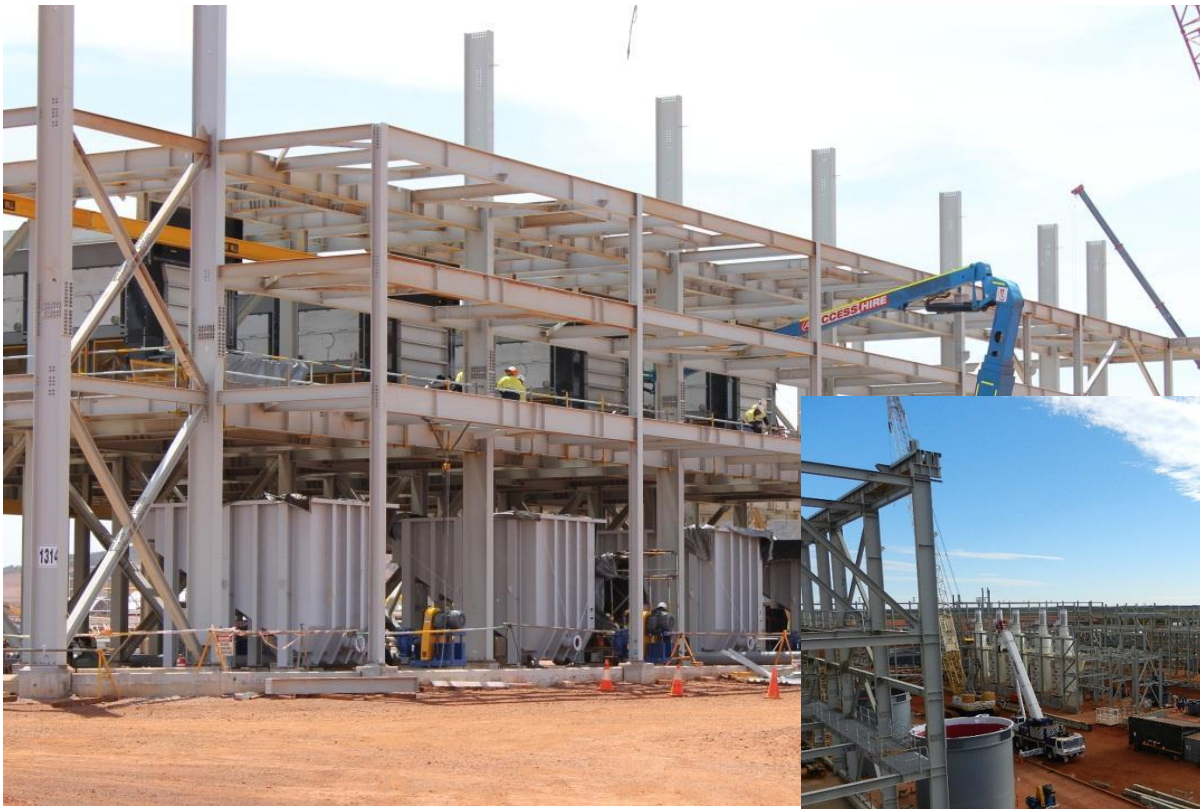
The Karara processing plant continues to take shape with structural steel, mechanical and piping work well advanced and electrical and instrumentation work underway.
