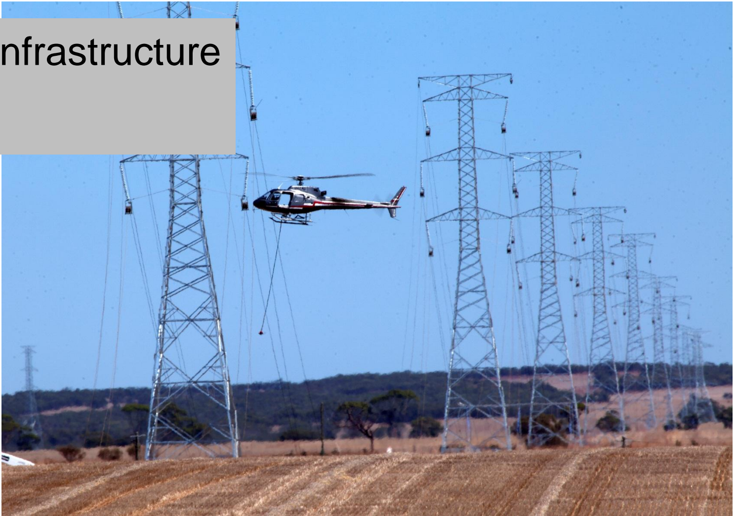
Aerial stringing of the 330kV power line is nearing completion.
