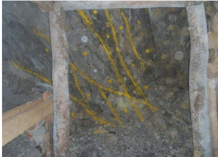
Sublevel 2 north 63mN face at end of the period.
