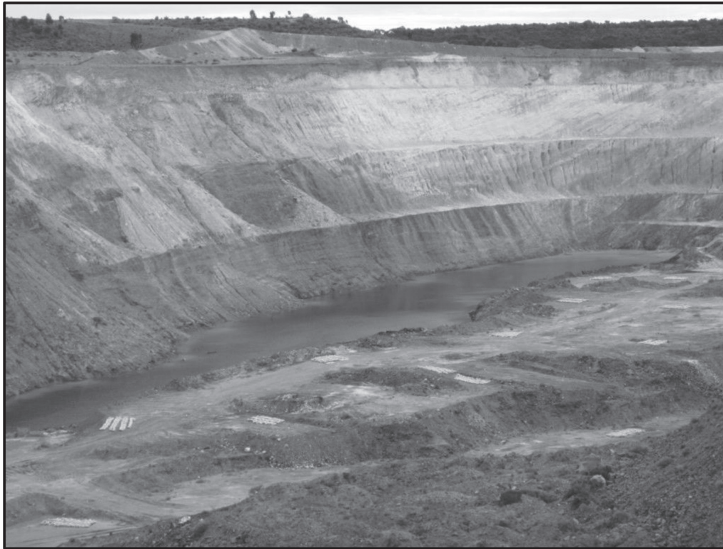
Figure 13. Bacchus pit looking Northwest where Laterite, Supergene and Primary mineralisation were mined
