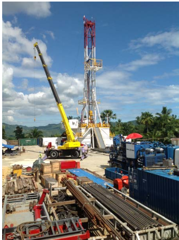
Jacob-1: Cementing Surface Casing (1 st November, 2012)
