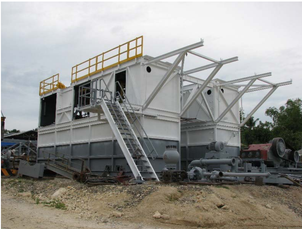
Rig-2: Substructure Undergoing Maintenance, July, 2012
