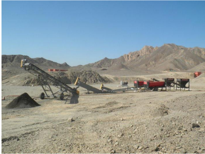
Alluvial Separator set up
