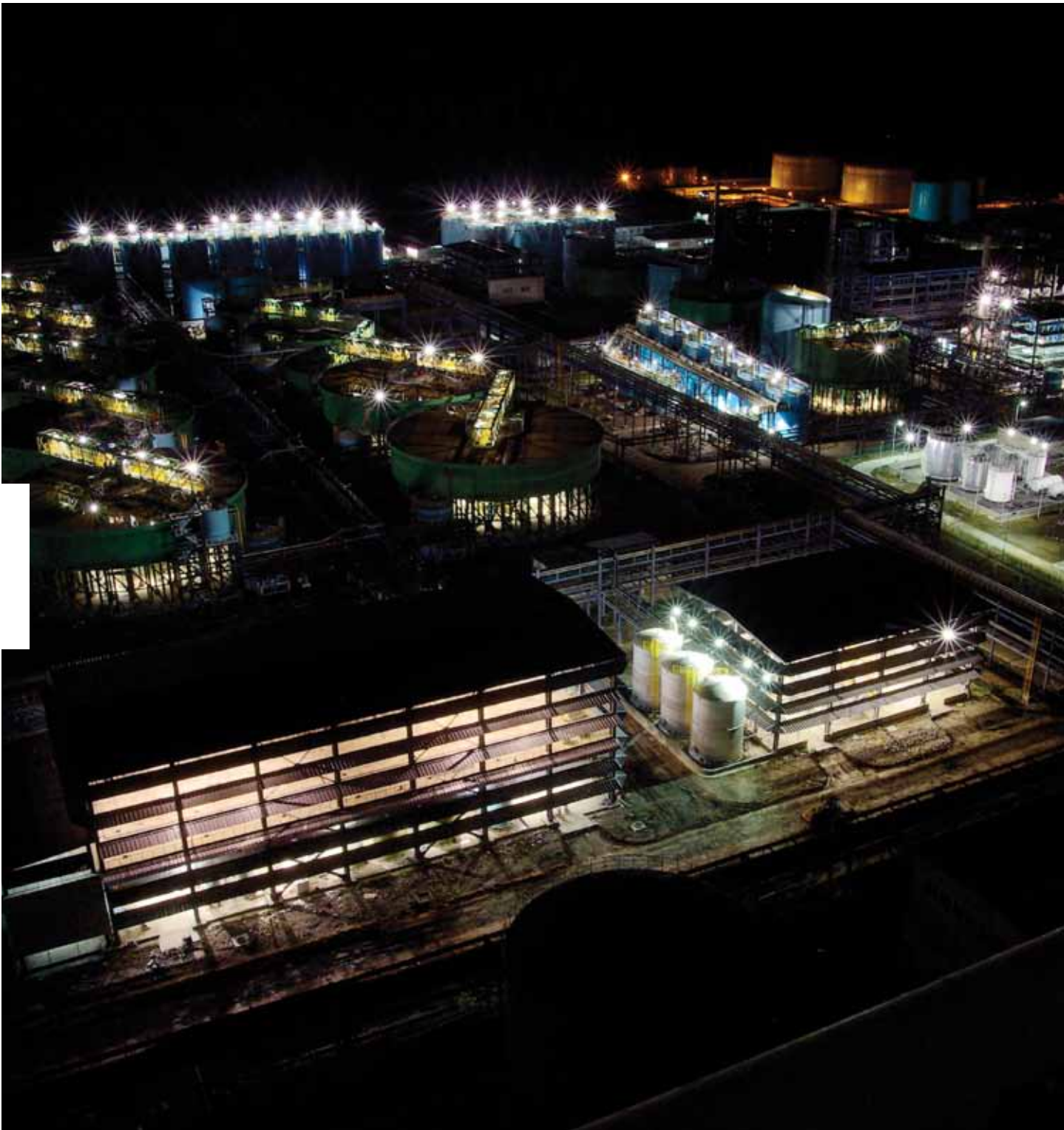
Ramu Mine - Basamuk Process Plant
