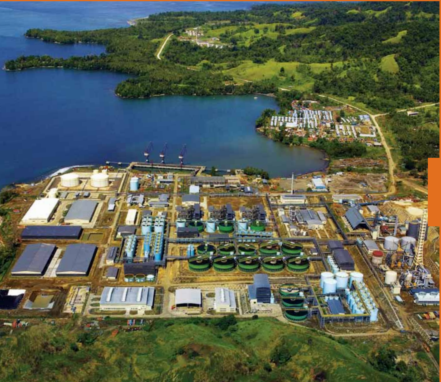
Basamuk Process Plant
