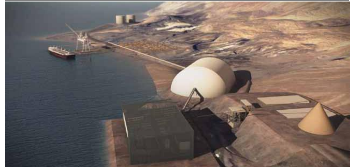
Process Barges with Concentrate Storage
