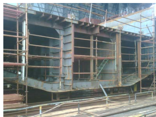
Figure 7: Construction of motorised barge
