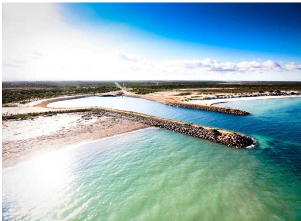
Figure 11: Existing Lucky Bay facility
