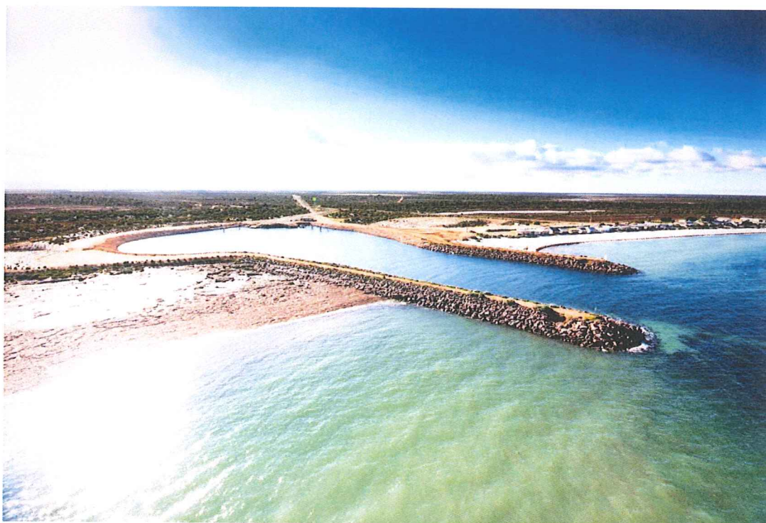
Figure 1: Existing Lucky Bay facility.
