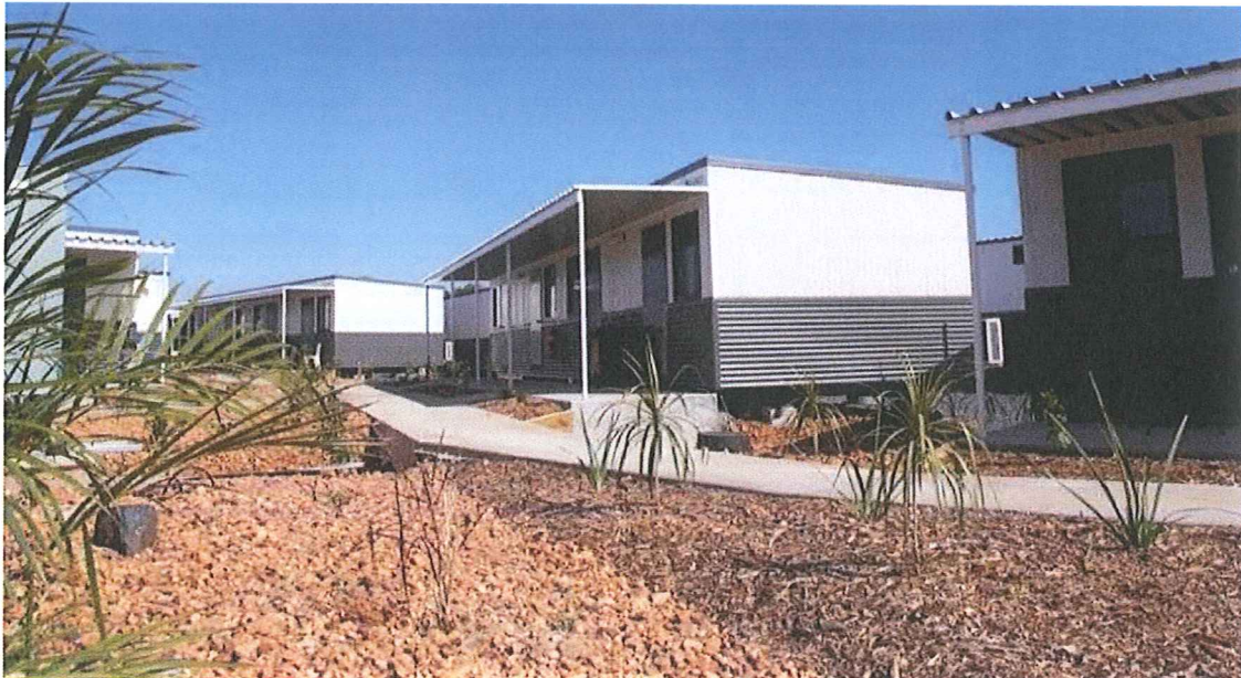
Figure 3: Accommodation village located in Kimba.
