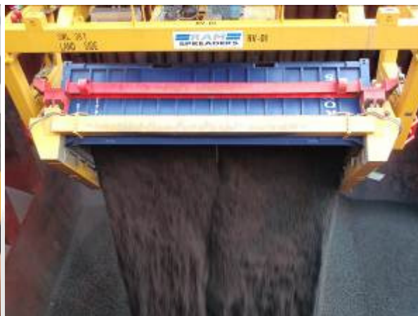
Figure 5: Rotating Spreader in operation
