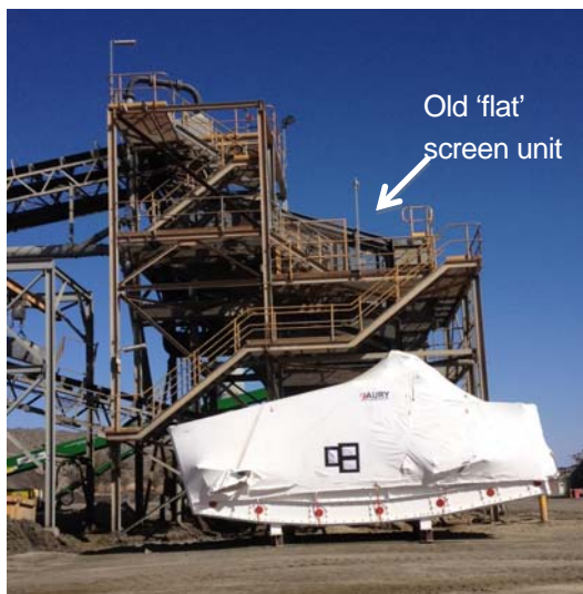
New 'banana' screen unit on-site and ready for installation.
