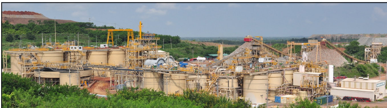
The Chatree plant site with the expansion plant at left
