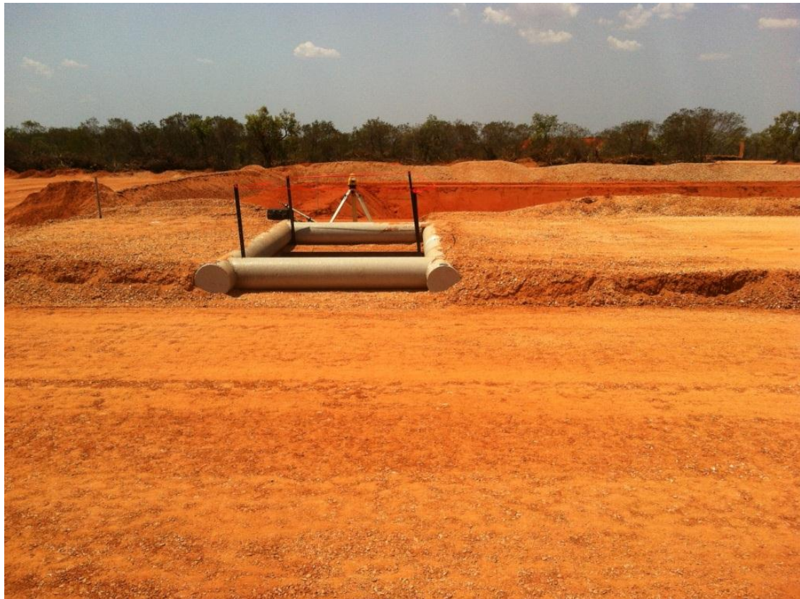
DCA Rig 7 drilling cellar (foreground) with sump (background)
