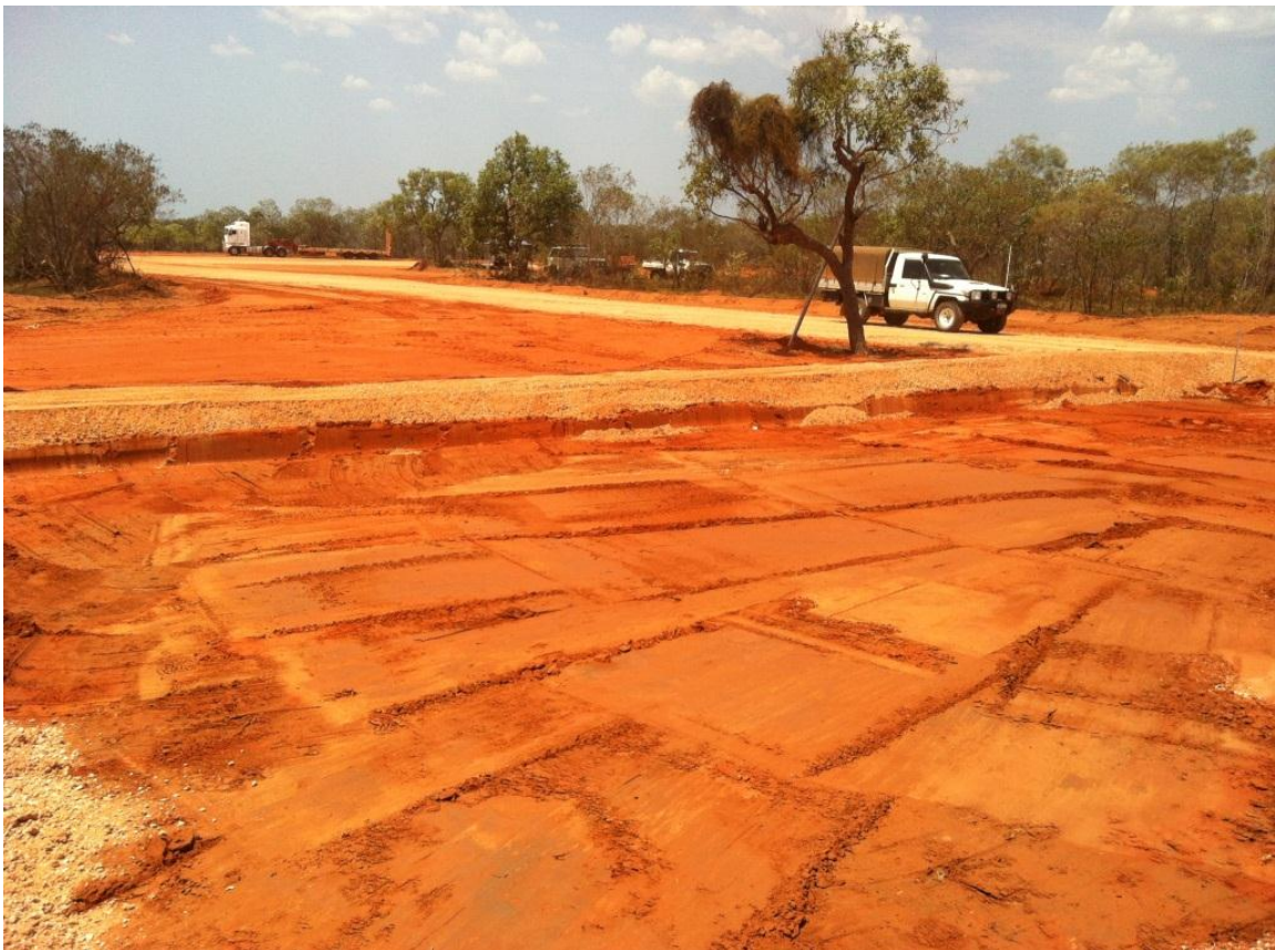
Graded roads into the well location and truck lay down areas
