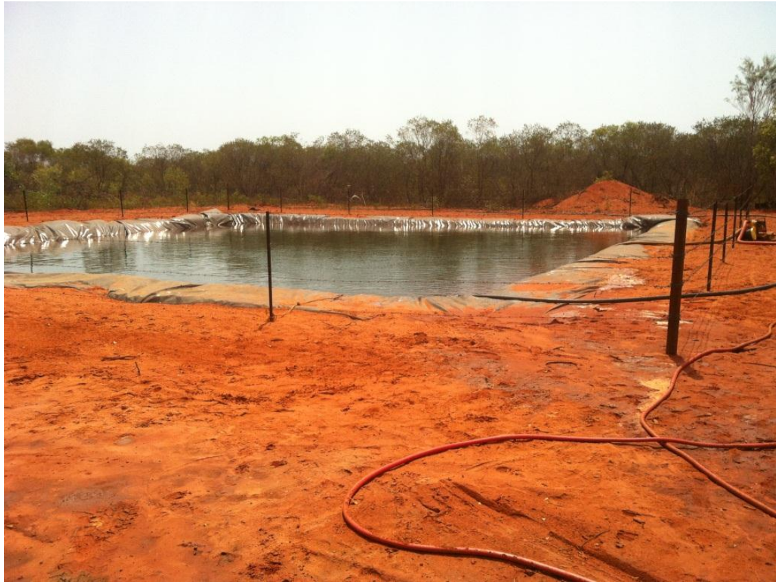
The Turkey's Nest located 40m from camp to provide water to Cyrene-1 operations
