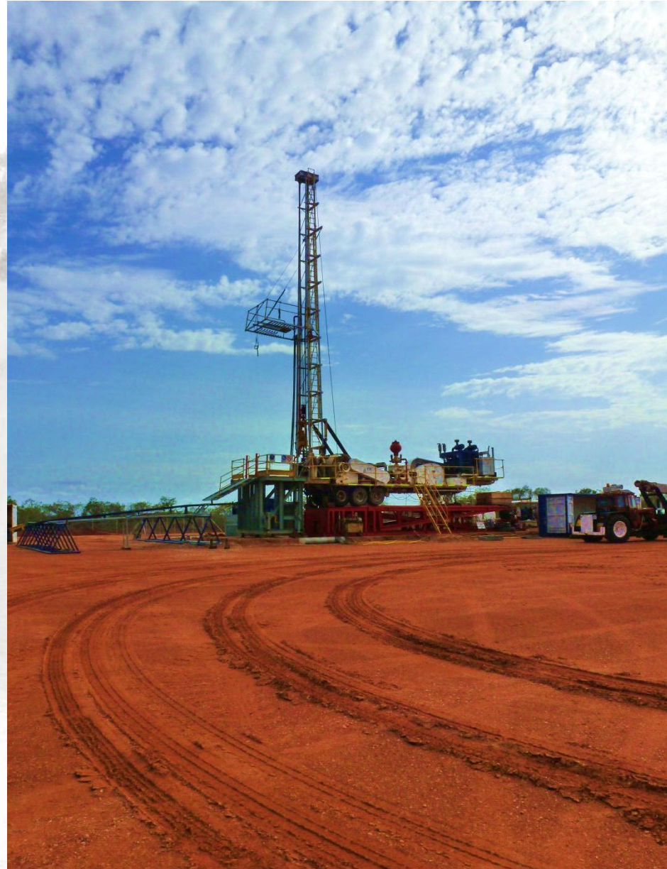
DCA Rig 7 rigged up on location pre-spud
