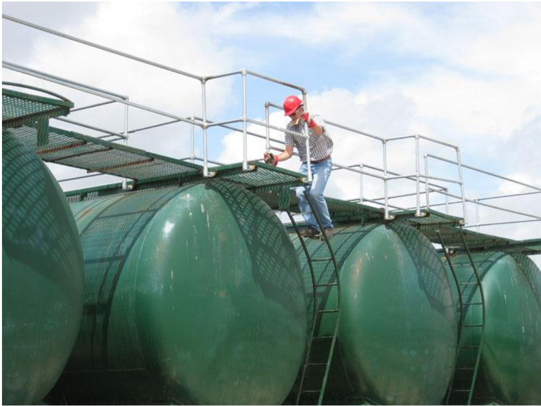
Tank farm Lidsey, Weald Basin U.K.
