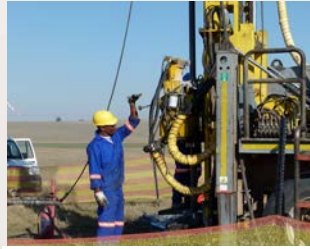
Coring rig operating
