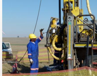
Coring rig operating
