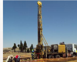
Drilling Hole KA-03
