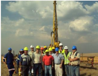
Commencement of drilling
