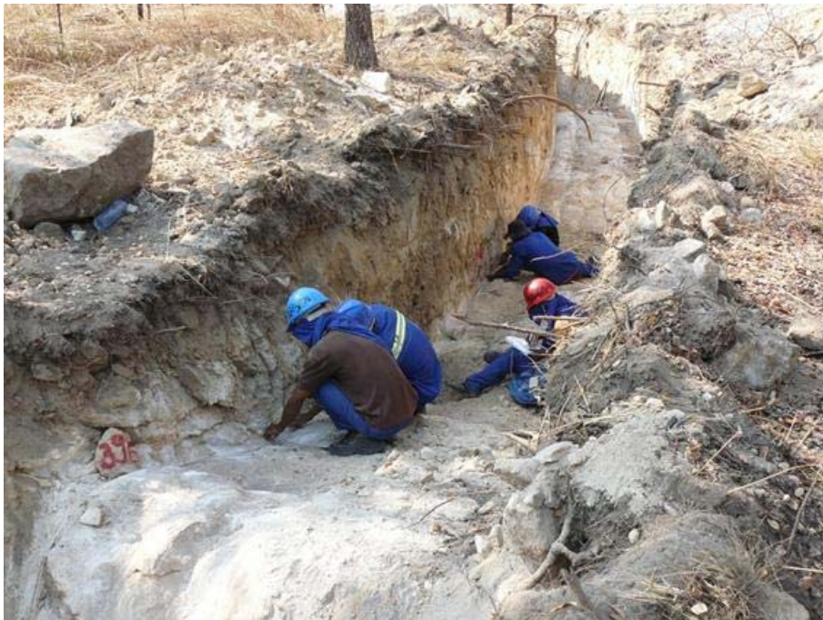
Figure 6: Trenching at Chigaio.
