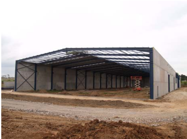
Progress on construction of the new facility in Smeaton Grange
