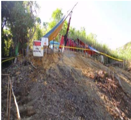
Sabang Prospect – drilling operations.
