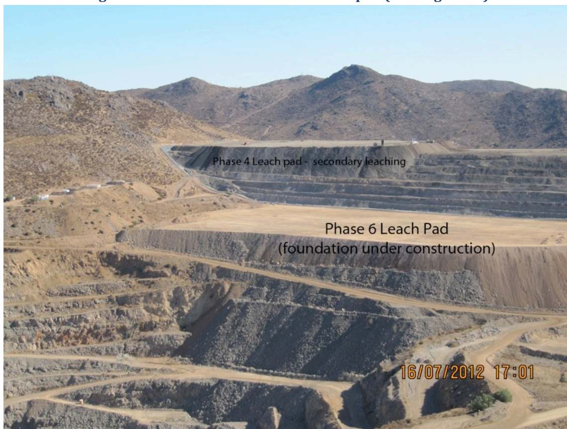
Figure 7- Construction of Phase 6 Leach pad (in foreground)
