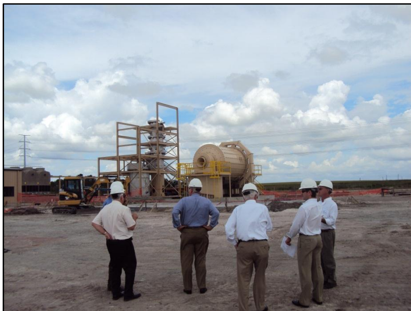
Figure 4: JDCP Demonstration Plant under construction September 2012
