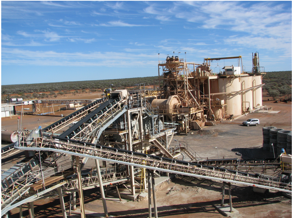
Figure 1: Existing Kirkalocka Processing Plant
