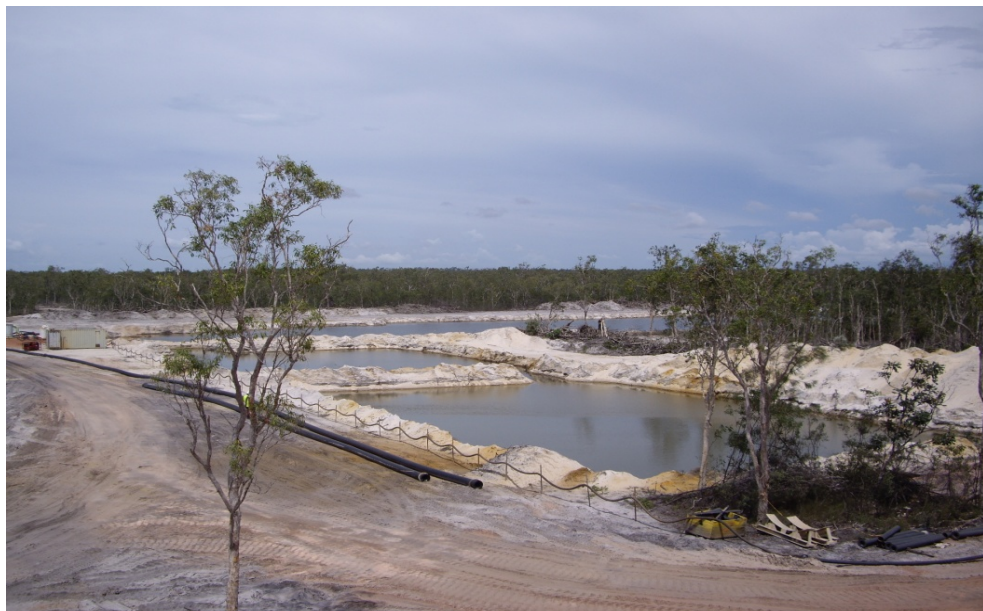
The plant water dams where water is stored and recycled into the processing operations
