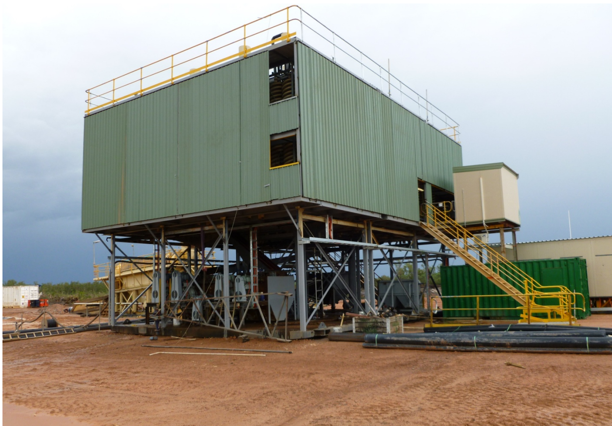
The Rebuilt Concentrator at Lethbridge South mine on the Tiwi Islands
