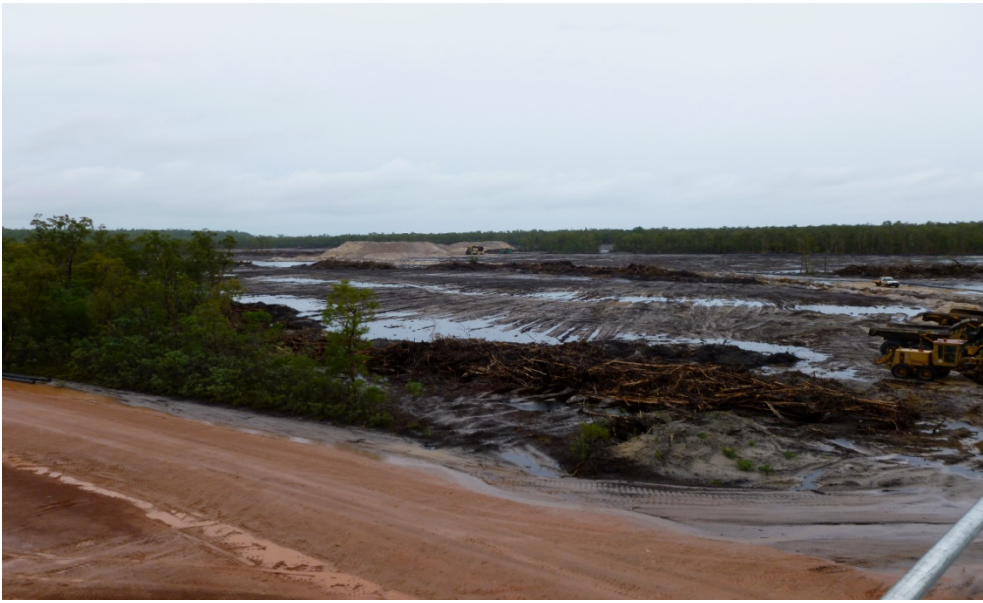
Part of the cleared ore body with the primary screening unit in the distance in front of stockpiled ore
