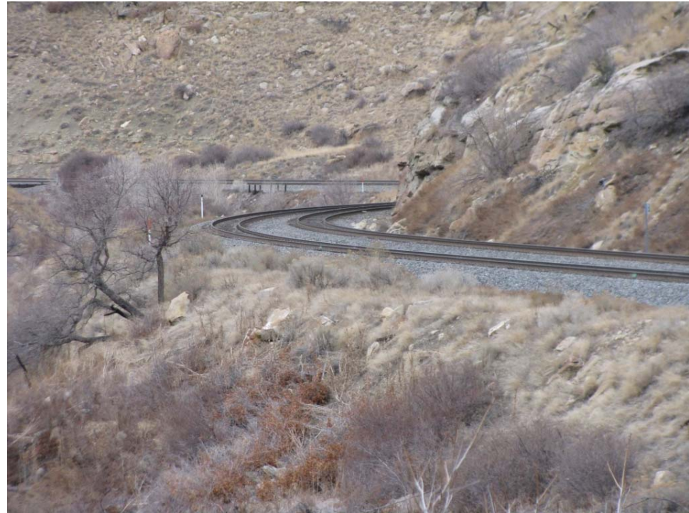
Dual-track mainline located less than 30km from Kinney Coal Project
