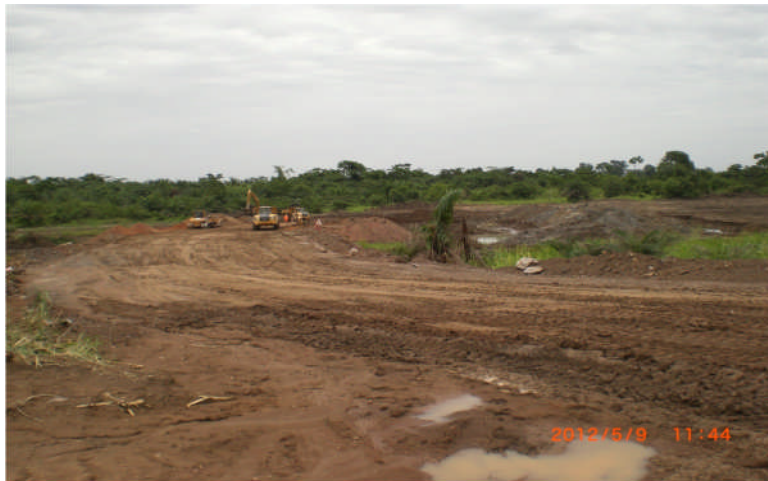
Old Tailings recovery operation - Levee 6
