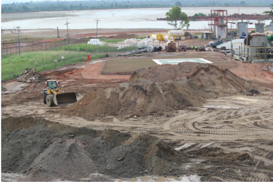
Ore and levee material stockpile for mill feed
