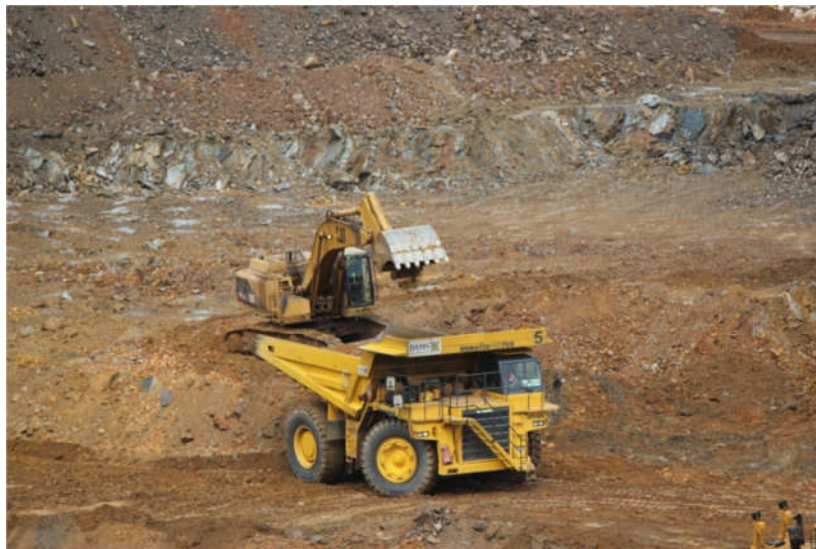
Strauss pit overburden removal post blasting operations
