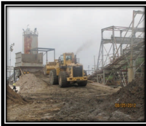
Loading the reclaim feeder
