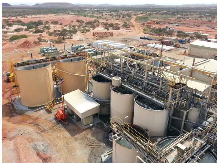
Figures 3 - New leaching tanks and Knelson Concentrator
