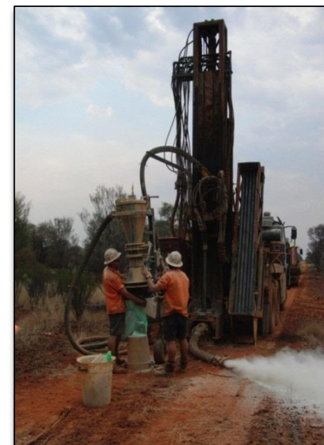
Drilling, Arganara Prospect
