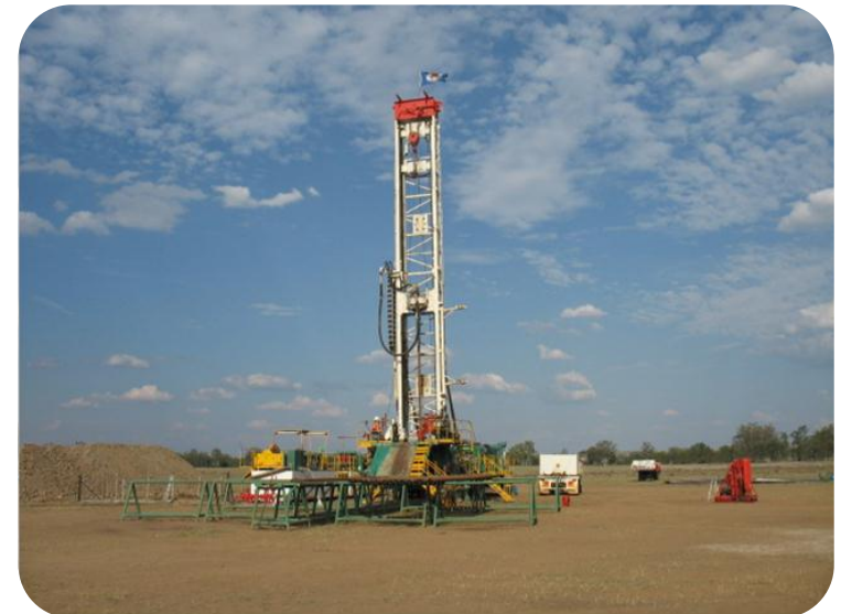
Dynamic Drilling Rig#17 East Bilna-1 (October 2012)
