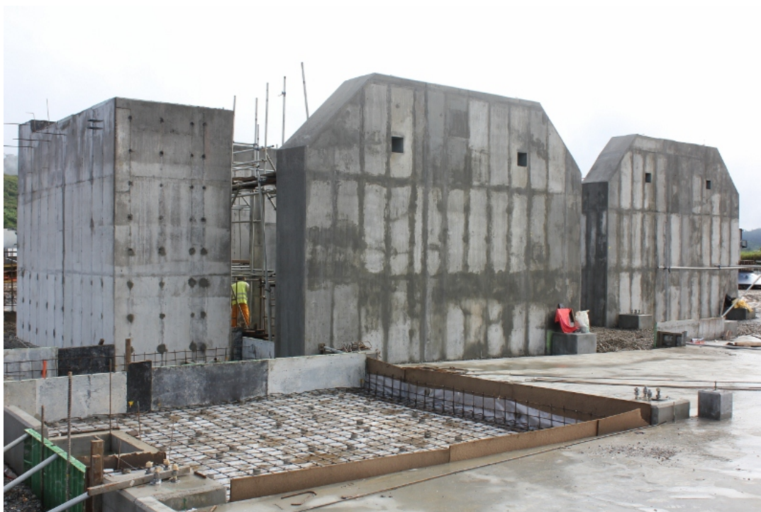
Figure 2: Completed grinding mill plinths, March 2012
