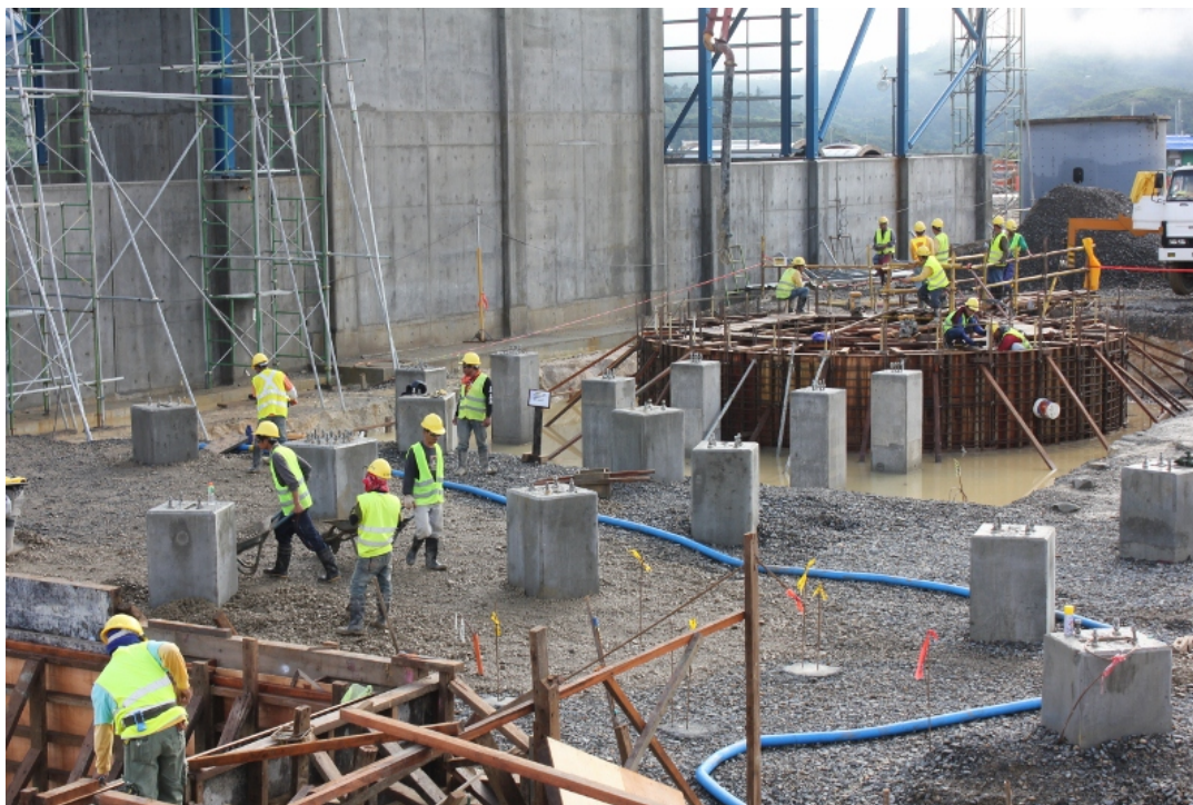
Figure 1: Concentrate handling ring beam, March 2012
