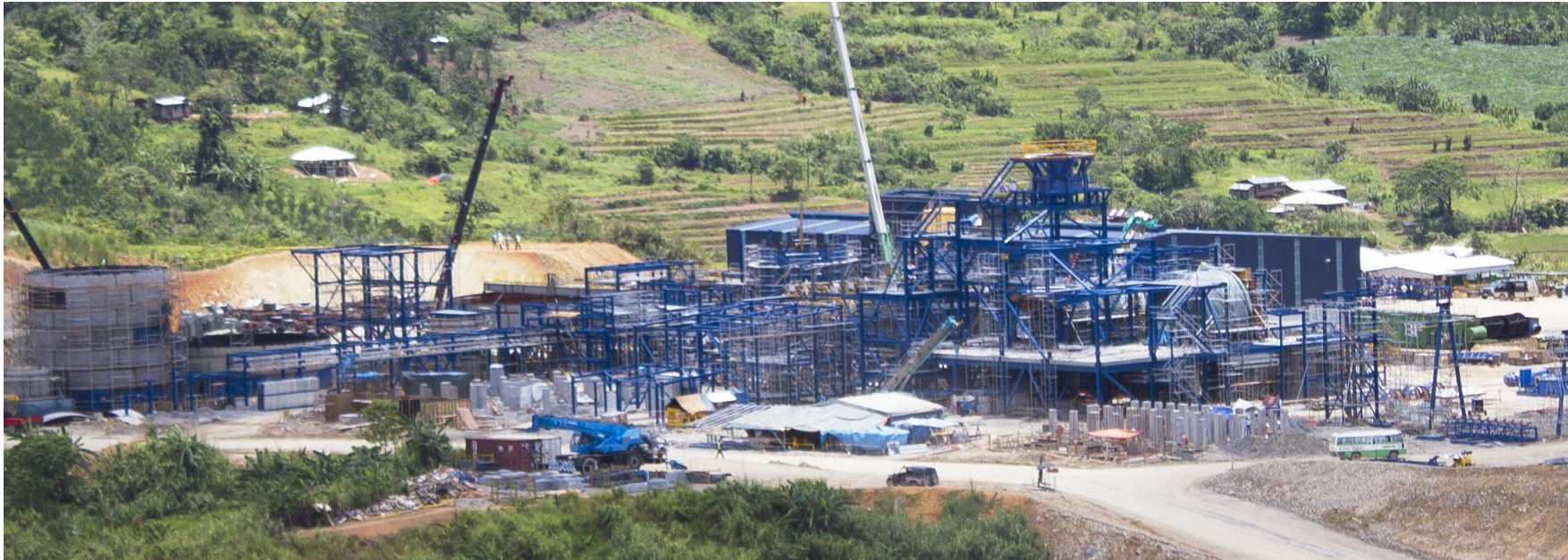
Plant site overview, July 2012
