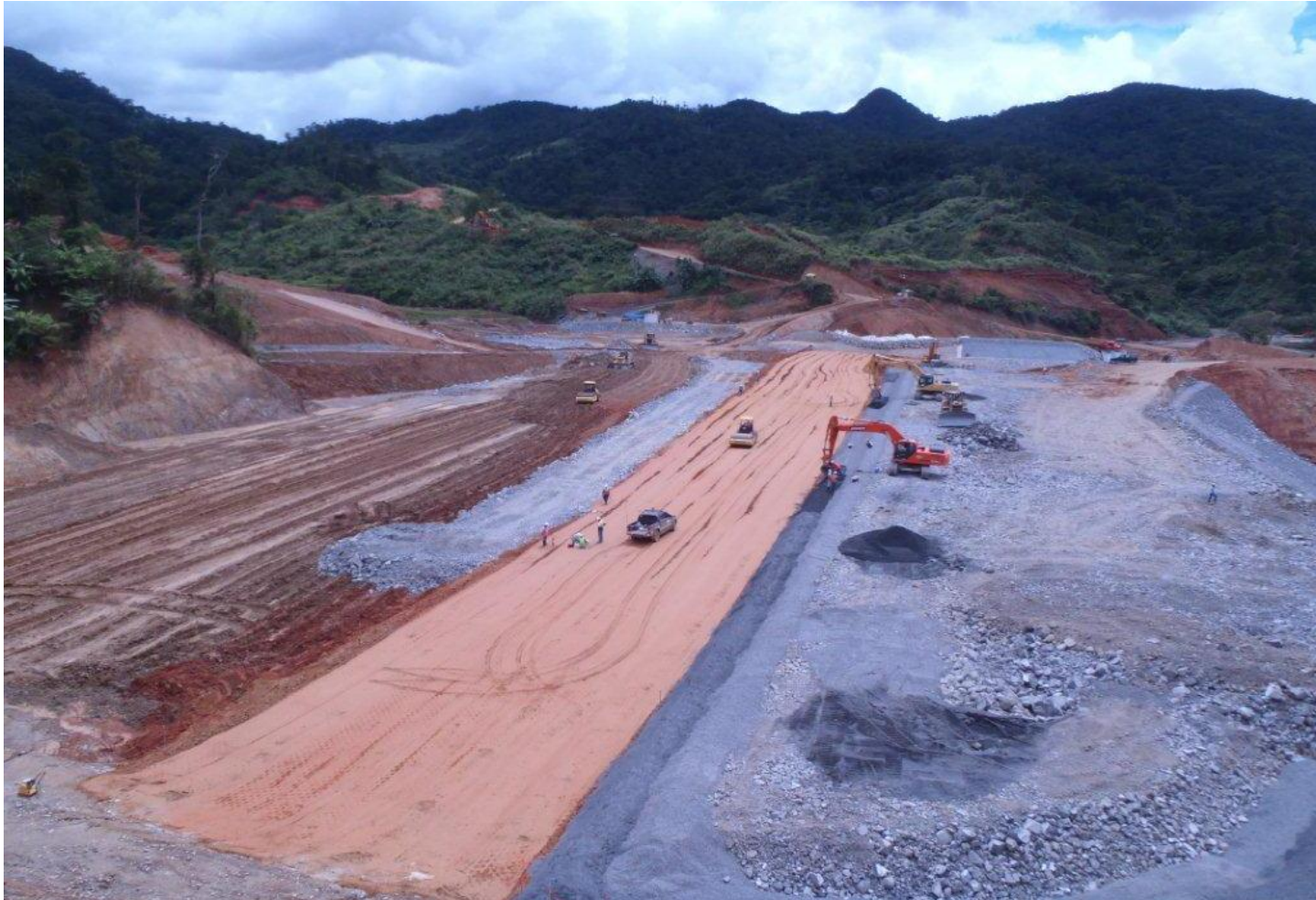
TSF construction 50% complete, June 2012
