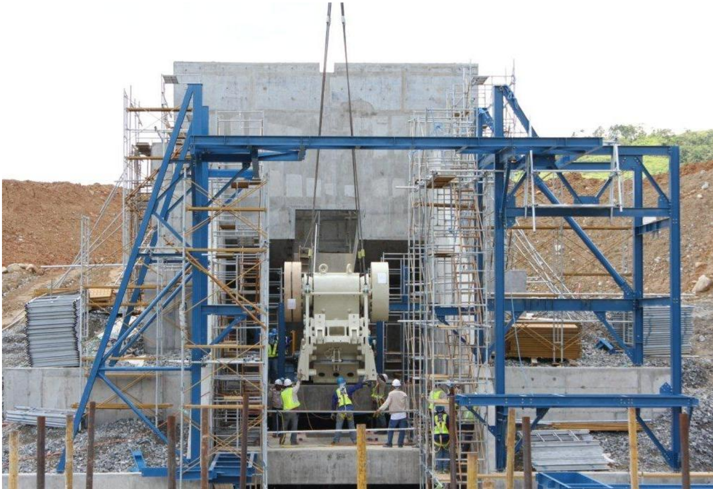
Installation of primary crusher, July 2012
