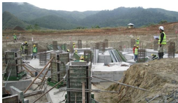
January: Tailings thickener foundation
