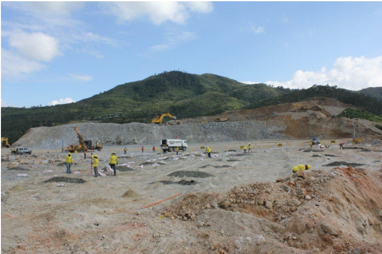
Figure 3 – Preparation for a blast at Didipio ore body
