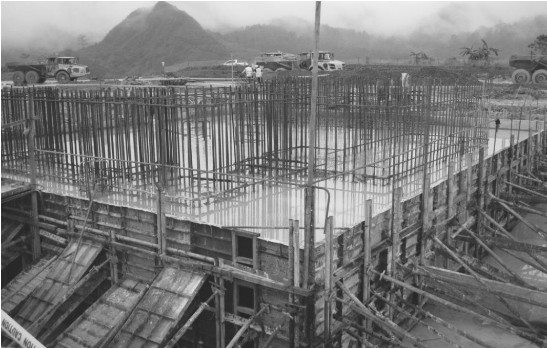
Figure 1: Completed concrete pour for ball mill base
