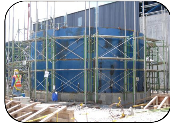
Concentrate handling tank
