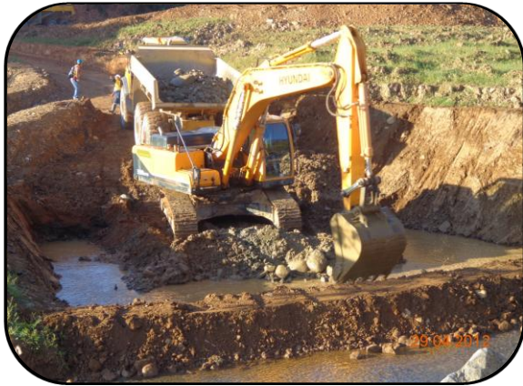
TSF construction of pump sump
