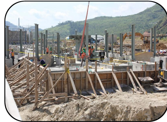
Tailing thickener concrete and steel works
