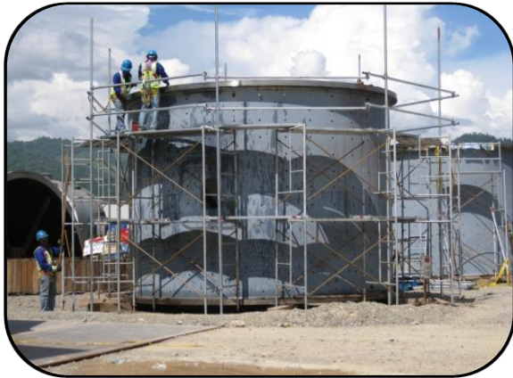
Cleaning of ball mill surfaces
