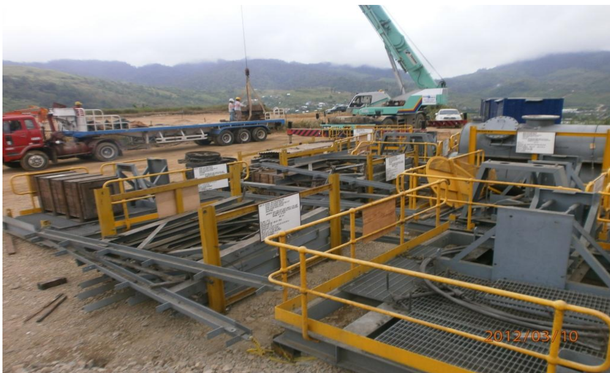
Figure 5 – Process Plant equipment being unloaded at site
