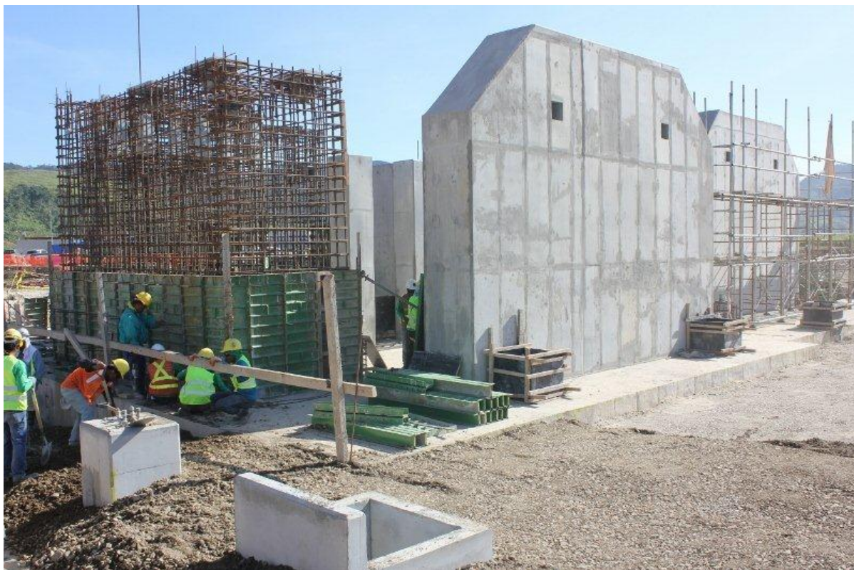
Figure 2 – Ball and Sag Mill plinth construction in progress
