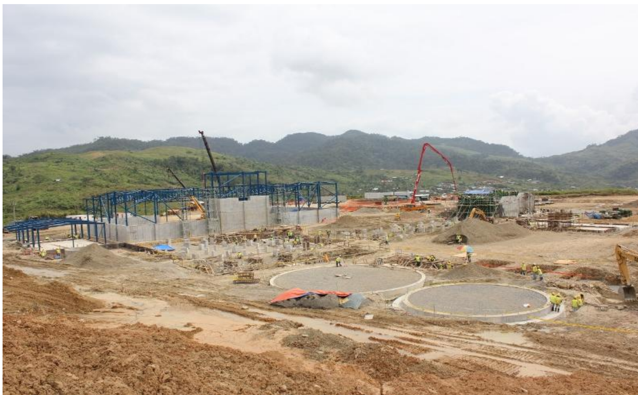
Figure 3 – Plant Site overview
