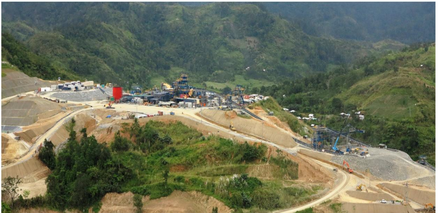
Figure 1: Overview of Process Plant, October 2012
