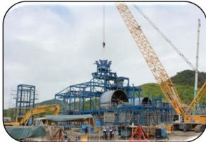
**Grinding Cyclone Cluster Erection**
