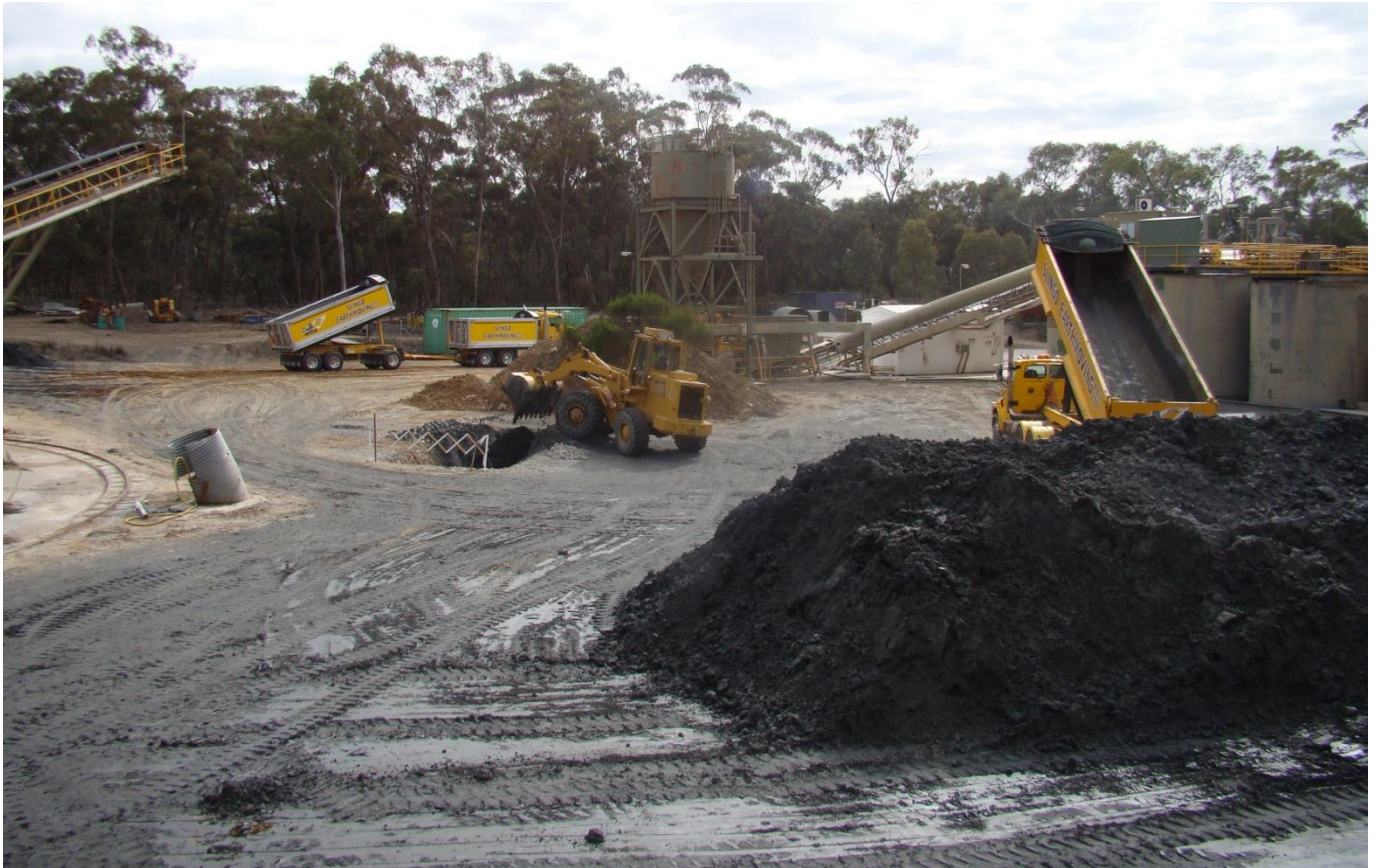
Tailings delivered to the Porcupine Flat Gold Processing Plant with loader feeding the ore shoot
