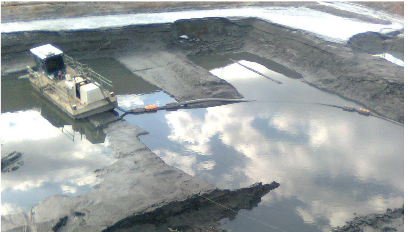
Example of a dredge removing tailings from a tailings dam
