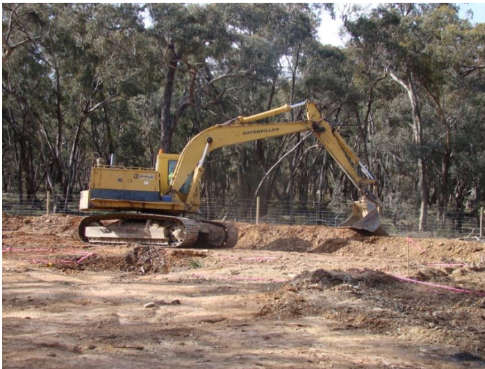
Construction of open pit bund wall
