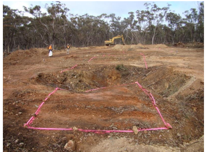
Top soil removed, sub-soil being removed, surface ore blocks in foreground
