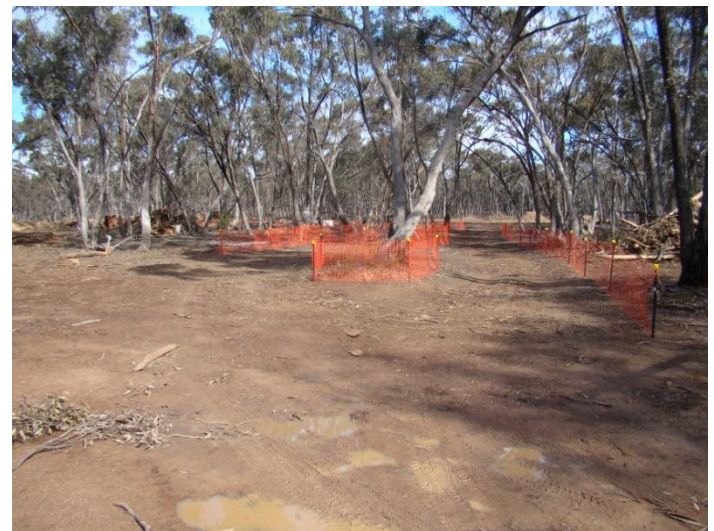
Barrier mesh being installed in mine area to protect vegetation
