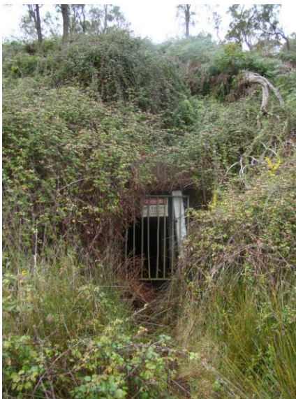
Entrance to Nuggetty Reef Mine adit
