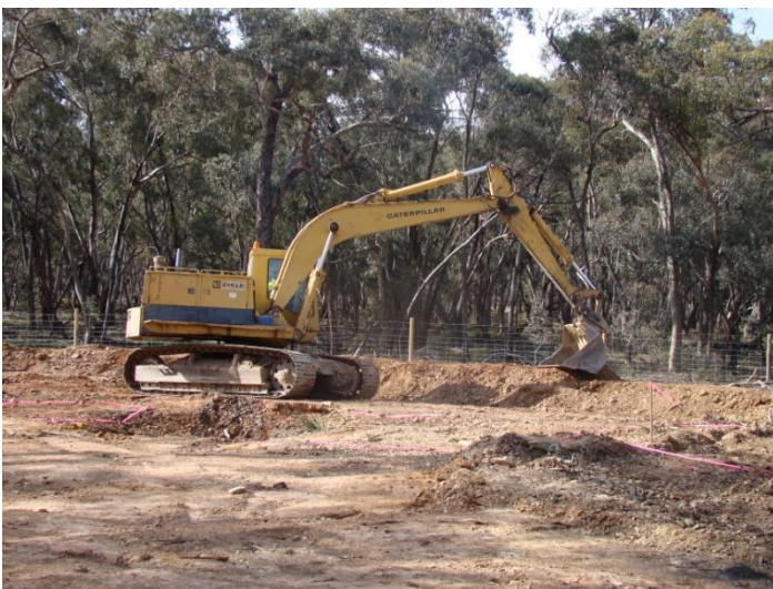
Construction of open pit bund wall
