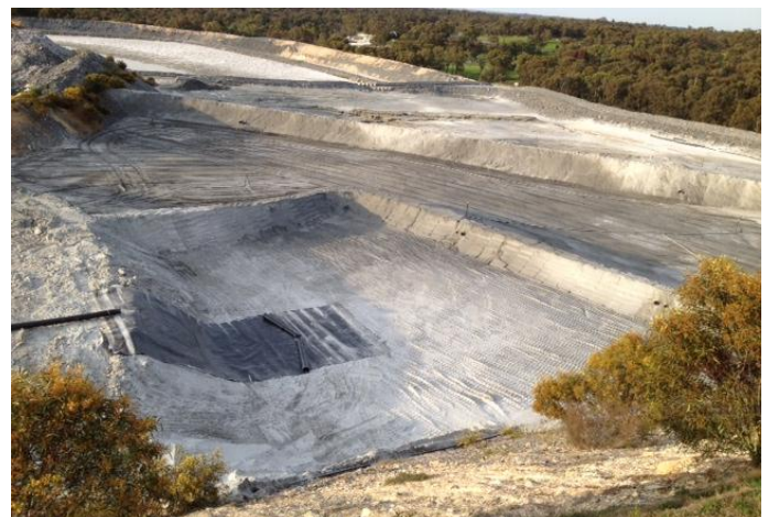
Prepared drying pads for Kangaroo Flat tailings
