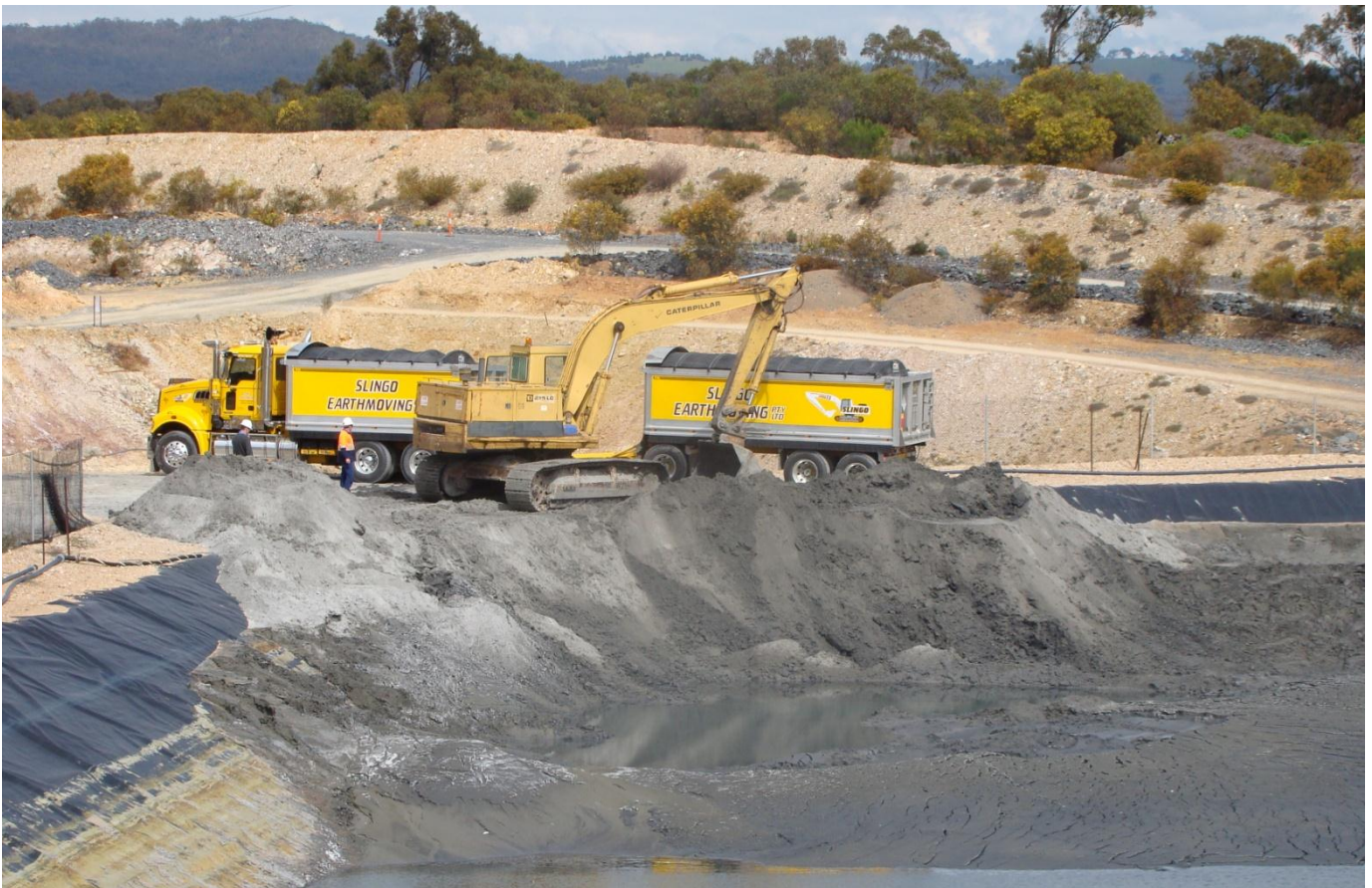
Excavator removing tailings from the Kangaroo Flat flotation concentrate tailings dam
