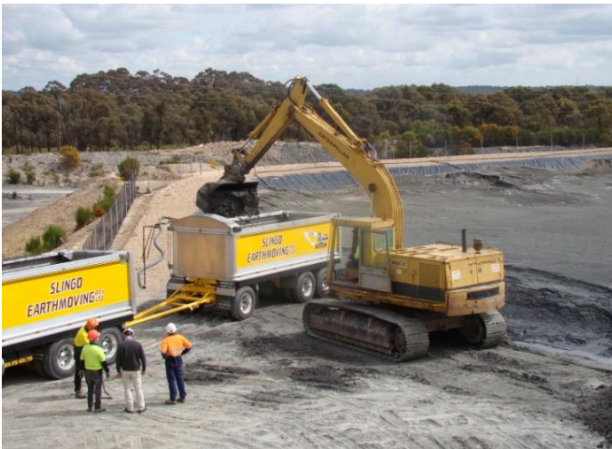
Excavator removing tailings from Kangaroo Flat tailings dam
