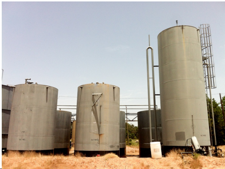
Catahoula Lake State # 22 production facilities (20% Otis)
